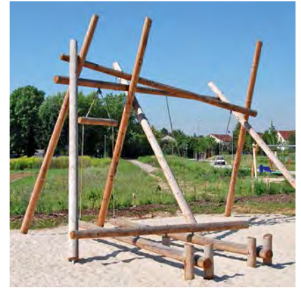
stand posts for swinging beams made of robinia
